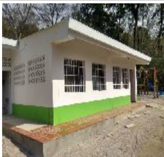
Vista General, Fachada Frontal
